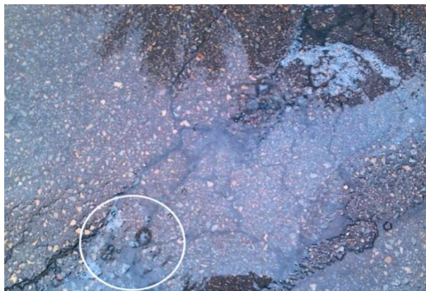
Fig. 2 Gas leakage spotted on the street
